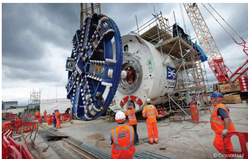
A tunnel boring machine (TBM) at the Docklands Limmo Peninsular Shaft in 2012
